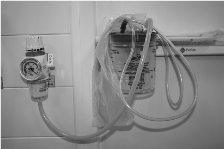
Fig. 5.5 Wall suction device.
